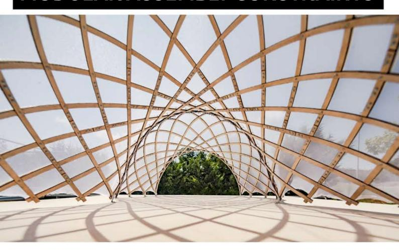
We'll work with flat collapsible elastic gridshells made out of straight planks to generate a large modular assembly. Workshop will run with Rhinoceros 3d Grasshopper
